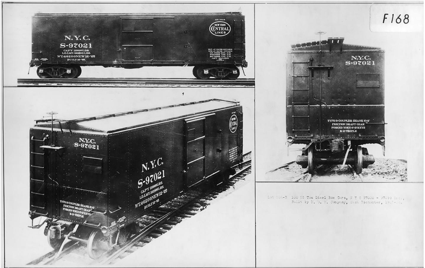
*New York Central East Rochester, New York shops builder's photos of the Lot 504-B box car. There are no visual differences between this car and the early PRR X-29 box cars. Note how the slightly longer wheel base in the design is evident in the side view. Photo courtesy of the New York Central System Historical Society.*
