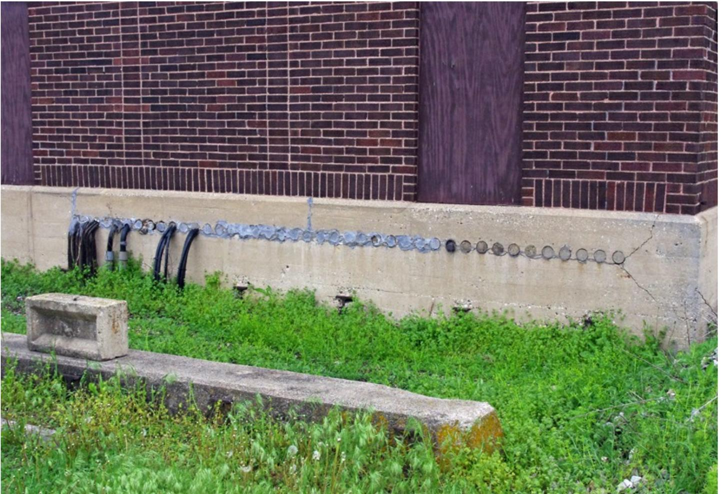
*This is the track side view of the Illinois Central tower at Ashkum, Illinois. The concrete in the foreground supported the square bars that came out of the holes in the concrete foundation. There were arms bolted to the square bars. When the bars were rotated, the arms pulled and pushed on pipes that ran to the signals and switches. Note the brick pattern at the sill and the square pattern on the wall. These details would show off your model well.*
