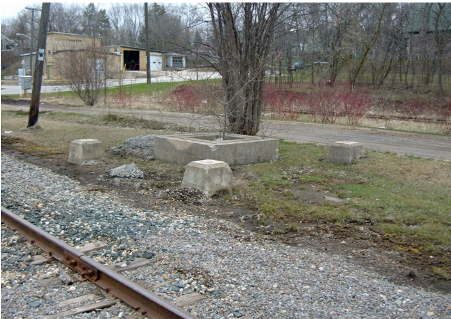
This is the foundation for the Milwaukee Road water tank in Plymouth, Wisconsin. The location of the four corners matches the tank in North Freedom, Wisconsin. You can also see the square form in the center for the frost box.
