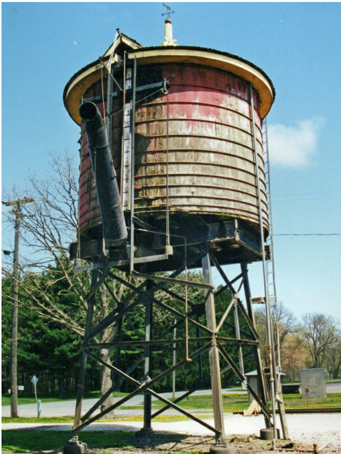
Another view of the water tank at the Mid Continent Museum. The tank was moved here, and when it was reconstructed they did not install the frost box.
