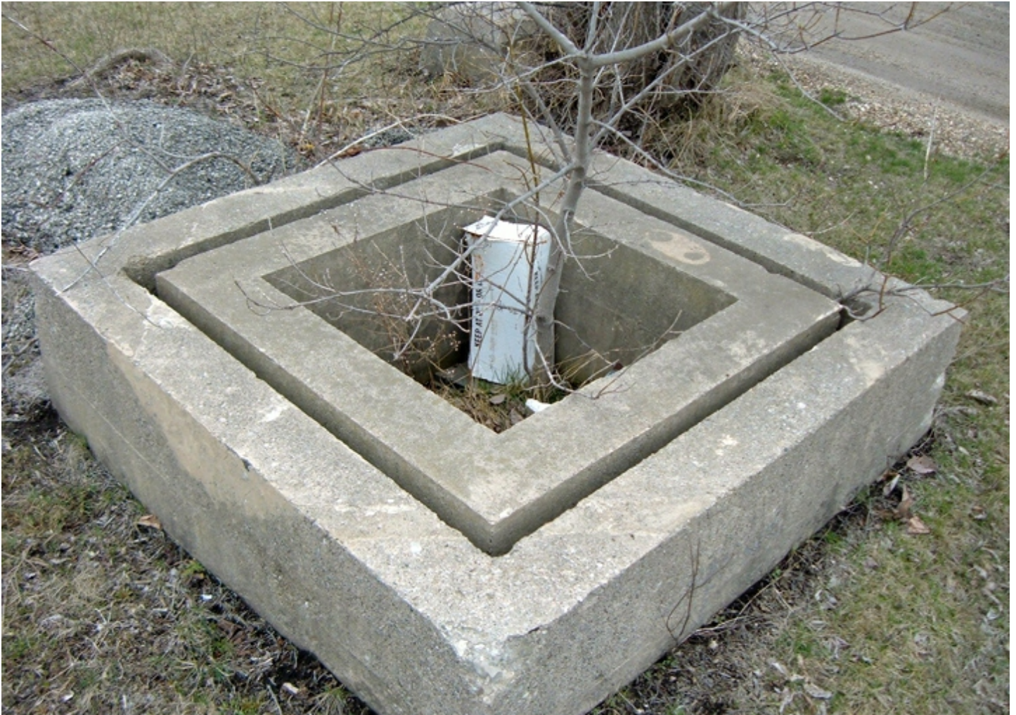
This is the base of the frost box for the Milwaukee Road water tank that was in Plymouth, Wisconsin. The water supply pipe would have been inside of the frost box to keep it from freezing in the winter.
