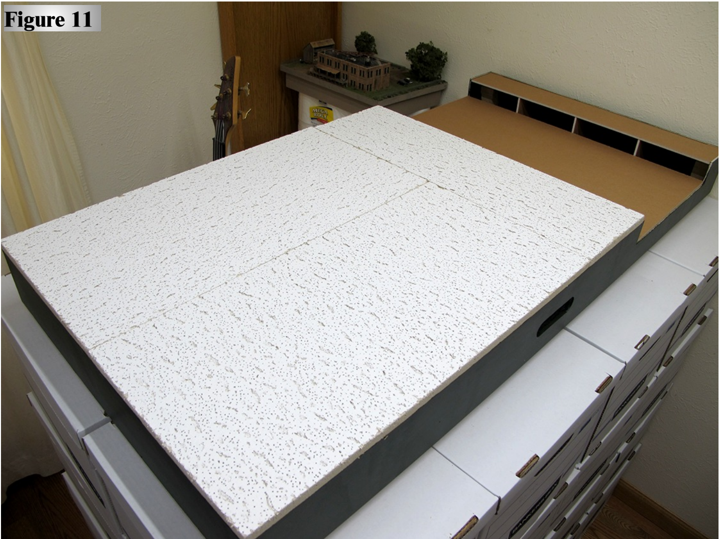
The module with 1/2" ceiling tile installed, for any additional sound-absorption, and possible vertical undulations.
