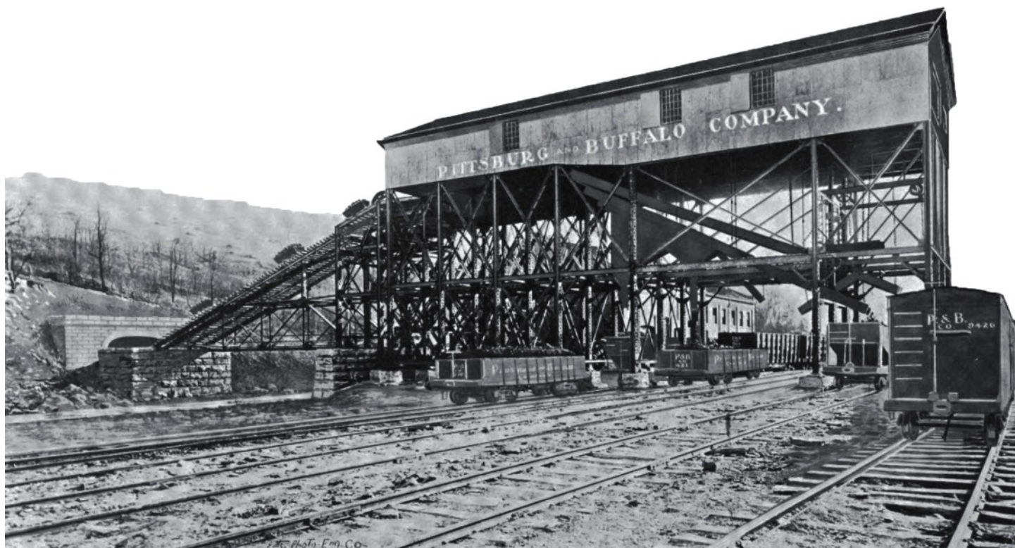
Page 281 of this Google-scanned 1901 journal has a photo of the Hazel Mine coal tippie, as built, in Canonsburg, PA
